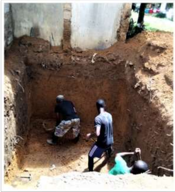
Left: Community and contractor digging the new septic tank
